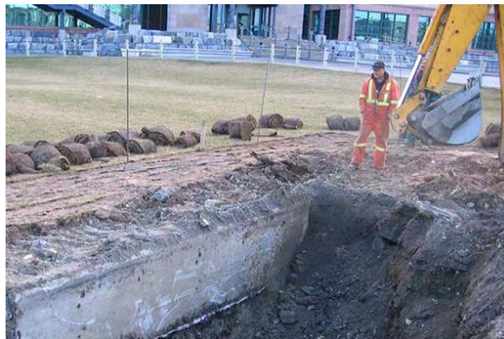
Portion of a concrete foundation and partial concrete floor uncovered at 'The Rooms' (Temple)
