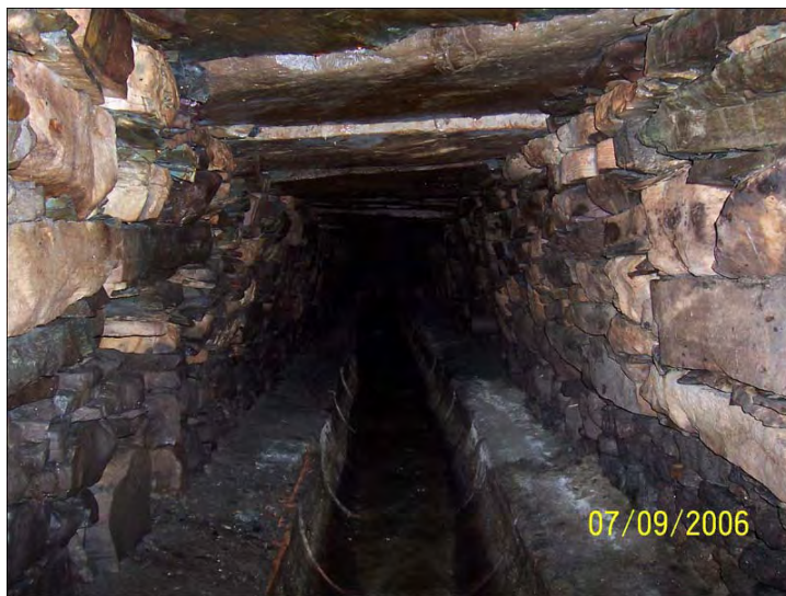
Interior view of 19th century stone sewer at Ayes Cove (Brandon Miller photo)
