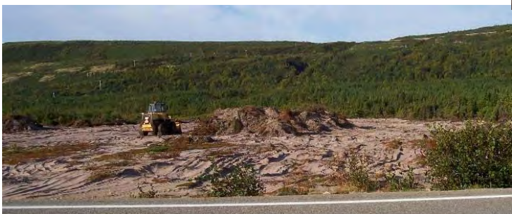
Damage done by front-end loader in L'Anse au Diable (Hull)
