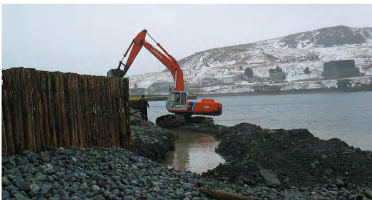
Hole #1 being excavated at the west end of the beach
