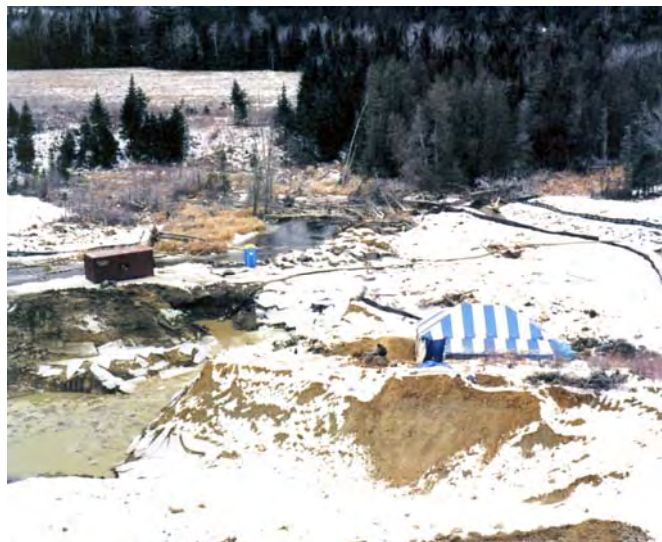
Excavation underway, under tent. Lower Guisiguit Brook in mid-ground, diversion ditch left of tent
