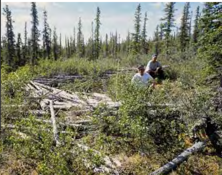
Collapsed Shya, Driftwood Hill Fence 2 Stephen Frost, Sr., and Joseph Bruce (R. Le Blanc photo)
