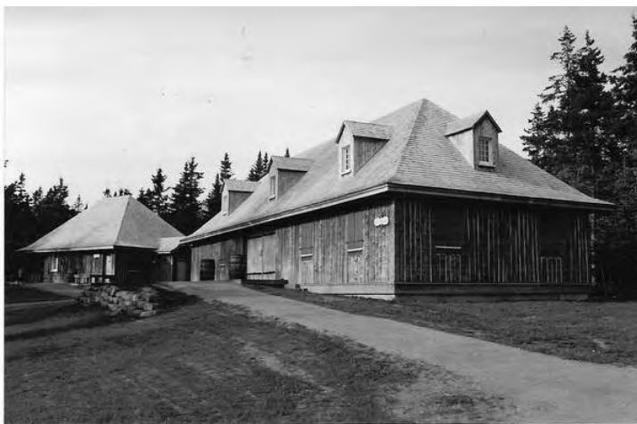
Public buildings at the Roma site on Brudenell Point, PEI, reflecting early 18 th -century French architecture
