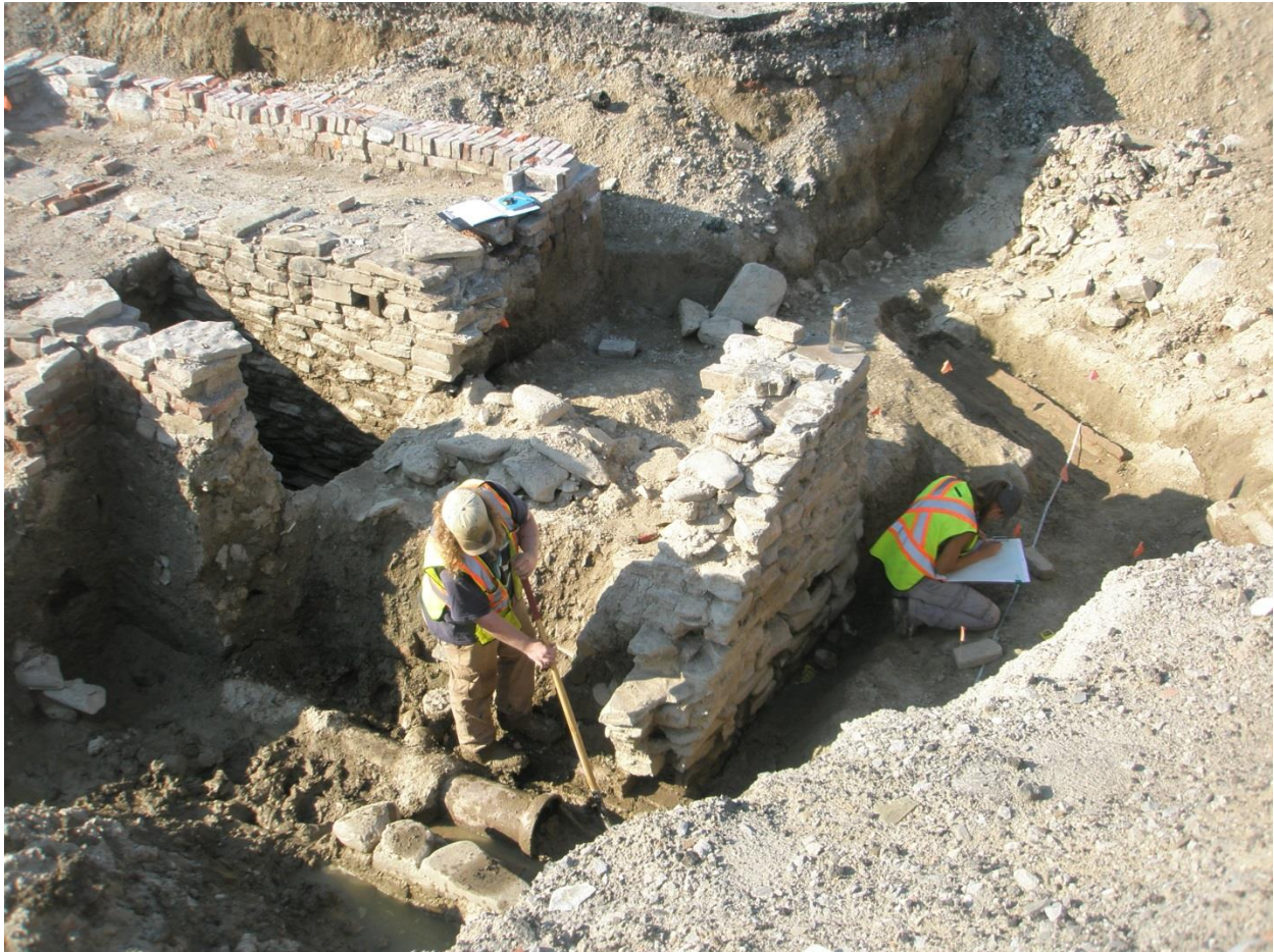
Figure 2. ASI's Chris Thorne and Kristen Hahne hard at work on the foundations of the New Fort Site (AjGu-32) at Exhibition Place (2013).
