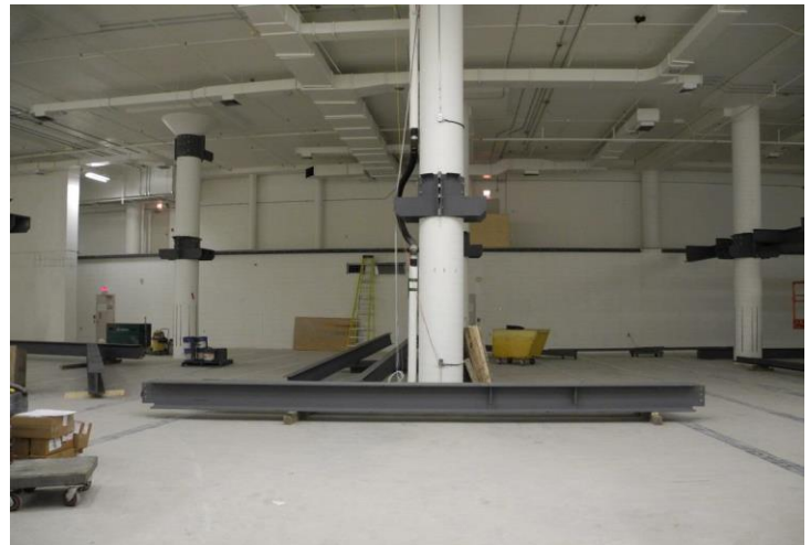
A beam inside Storage Room 5103 awaiting installation.
