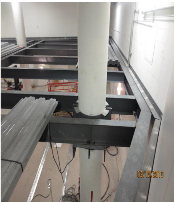
Metal angle beam attached to perimeter walls to support floor.
