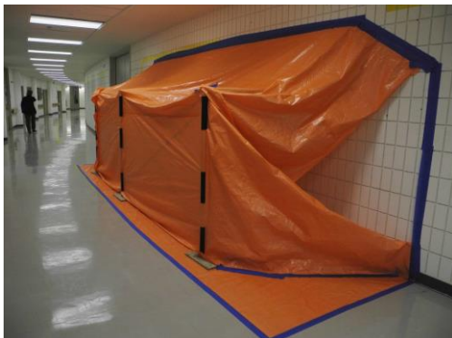
Section of corridor wall removed for beam entry.
