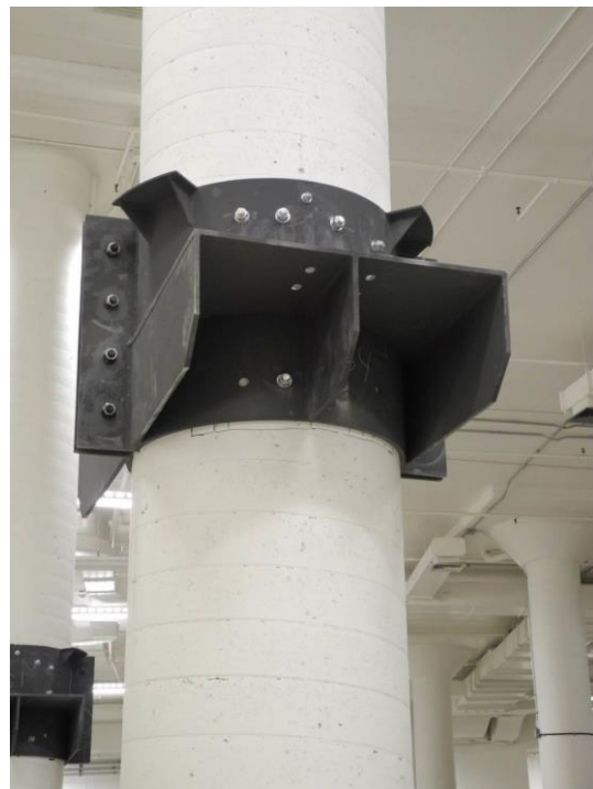
Installation of metal collars to support the steel beams.
