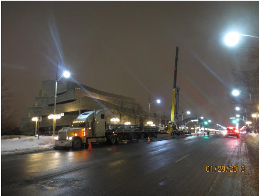
Delivery of the beams started on a cold and rainy night.
