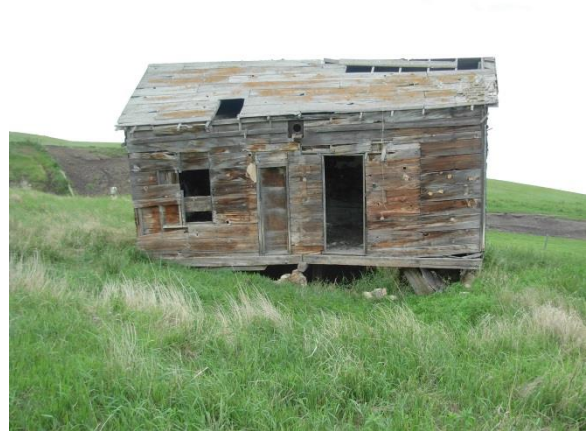
Figure 8. View of southeast wall of standing structure at FaOp-75.
