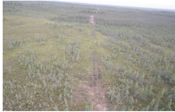
View northeast of E - D crossing/cut, muskeg meadow.
