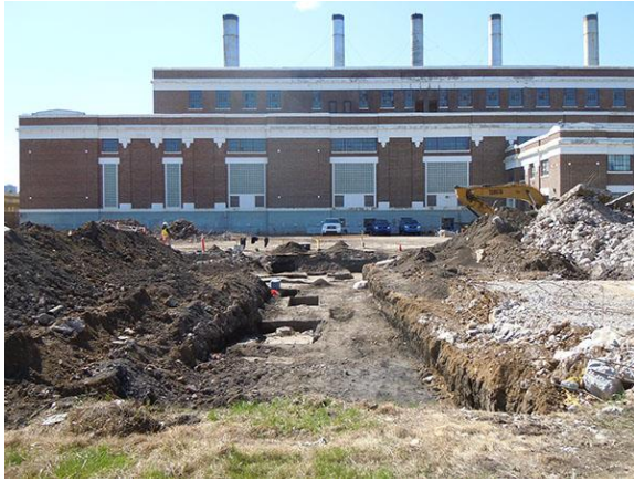
Figure 3. View of excavation block on east side of EPCOR's Power Plant.
