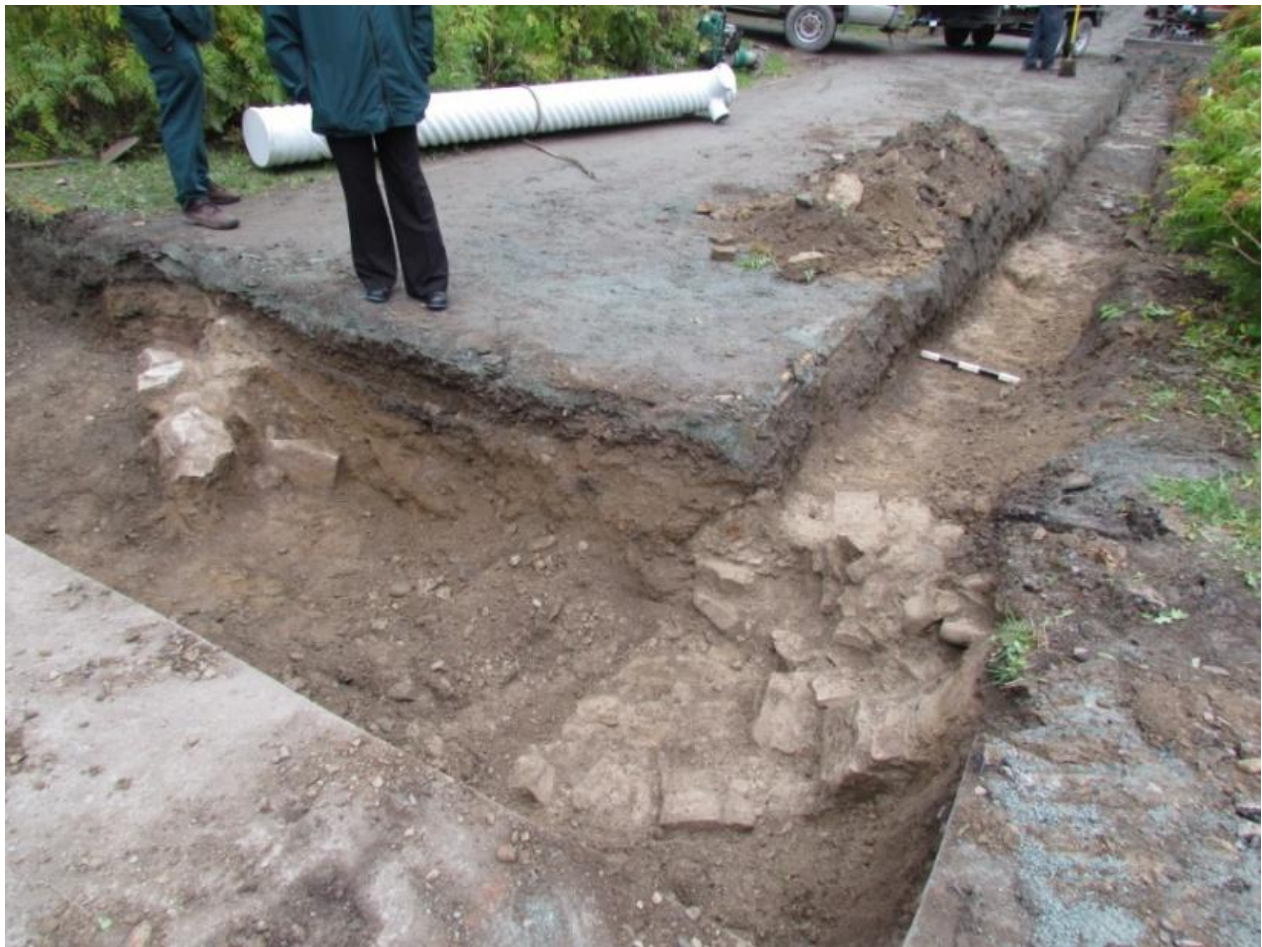
Foundations of the seigniorial mill (17th century) uncovered during drainage work.
