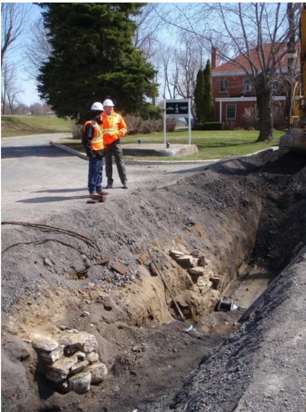
Remains of the stone foundations of the barracks built in 1790 and uncovered during the dig in spring 2011.
