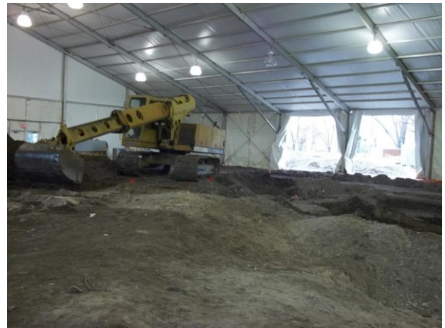
Figure 6. Mechanical removal of imported fill.
