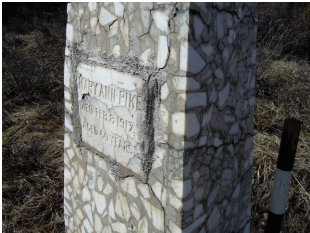
Figure 1. View of the name plate of the Mary Ann Pike monument in Mountain Park Cemetery. Note cracking and spalling of weathered marble plate. Previous attempts to fix the plate with incorrect materials may have accelerated the degradation. Cracking between marble terrazzo pieces of obelisk-style monument is also a concern.
