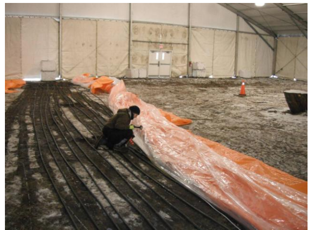
Figure 3. Laying out ground thawing hoses inside tent.
