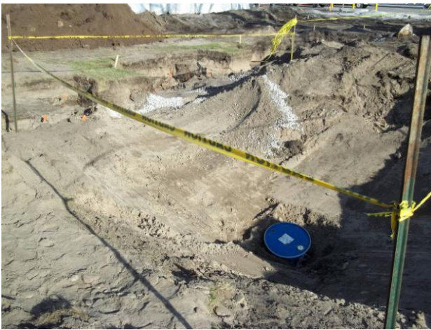
Figure 11. Installing perforated drum in sump pit.
