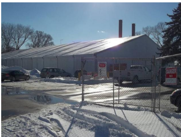
Figure 1. Tent used to cover majority of site area in winter.
