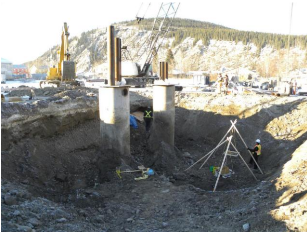
Dawson Wastewater Treatment Plant excavation. Coffin under plywood in back corner of excavation.
