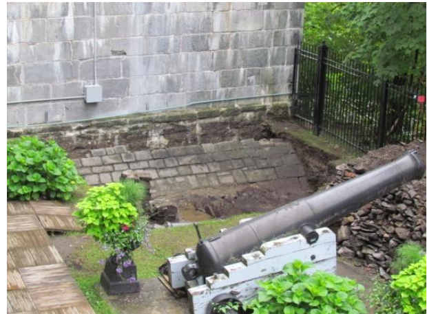
Gutter built in 1846 in front of the escarpment on the right flank of the Governor General's bastion, partially destroyed during work in the 1900s.
