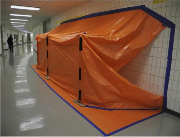
Wall section removed to permit the transport of large steel beams into Collections Room 5103.
